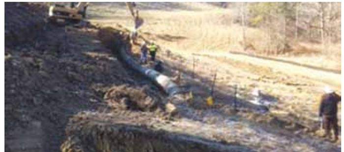
Our IMU data analysis identified a pipe that had been displaced 10 ft. downhill, with a bending strain >1%. Failure was avoided.
