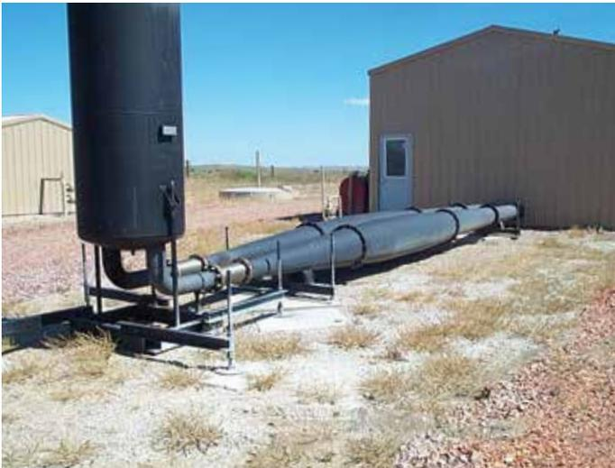
The length and shape of the pipes controls the process of scavenging and trapping fresh air in the power cylinders.
