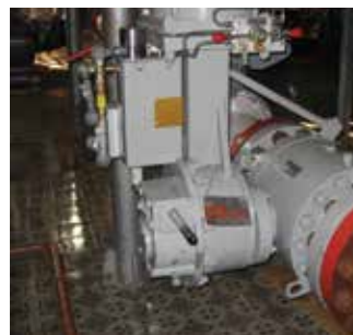
Figure 2 - Control valve installation AFTER installing ANJ
