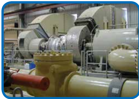
Figure 9 - Surge Control Valves Centrifugal Natural Gas Compressors (Natural Gas Transmission Industry) Becker Surge Control valves provide increased protection for centrifugal natural gas compressors. The Surge Control Valve will open rapidly upon potential surge to protect the centrifugal compressor mechanism. Becker Surge Control Valves are well accepted by many natural gas transmission companies and natural gas compressor manufacturers throughout the industry. For additional information see Becker’s Surge Control Valve Brochure (SCV)..
