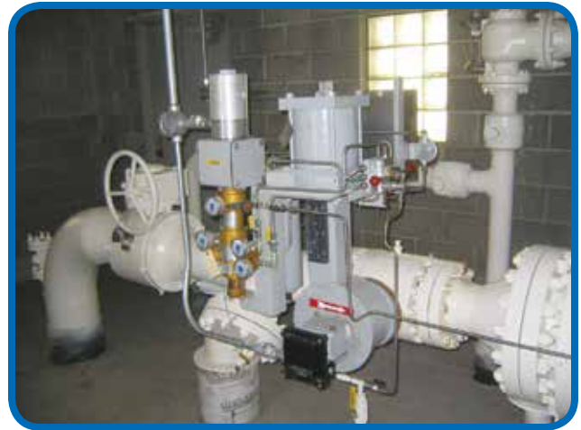
Figure 2 - Becker RPDA Actuated Control Valves
