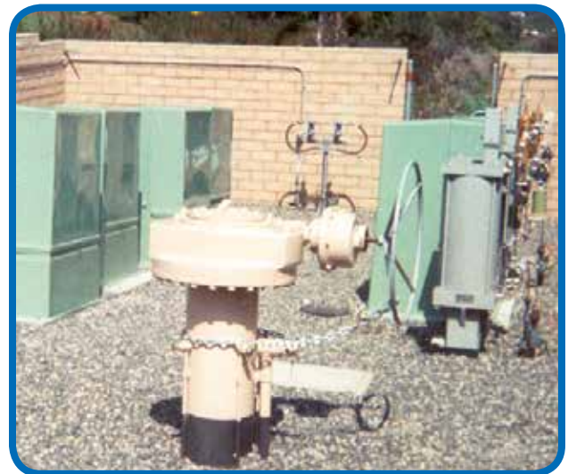
Figure 12 - Installation of Becker Below Ground Regulators (After Backfill)
