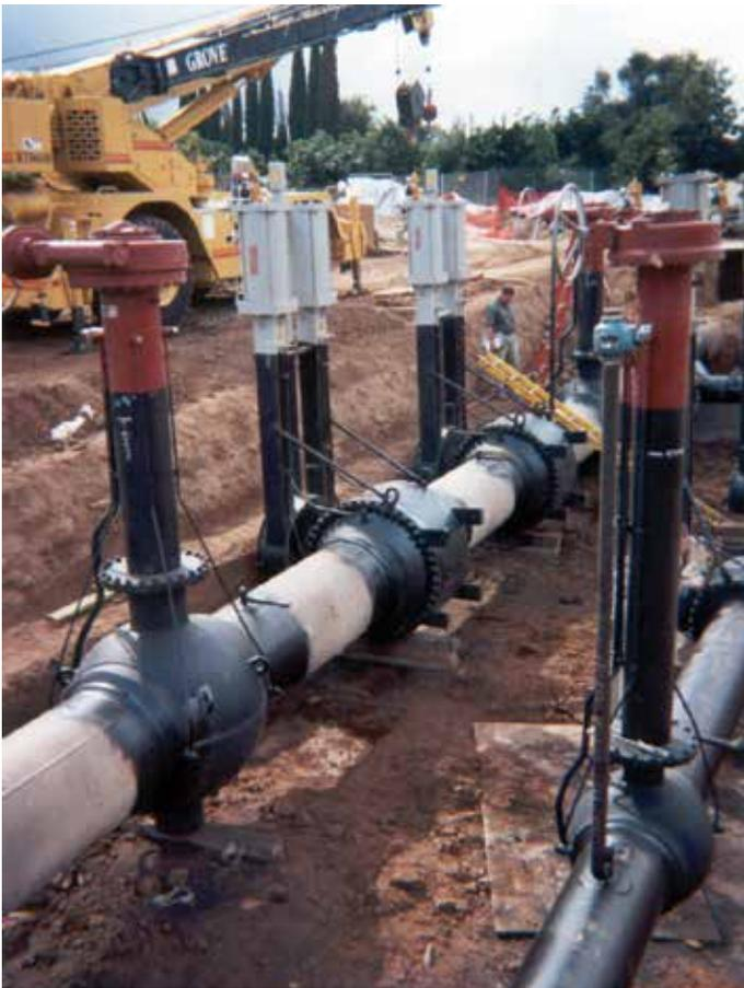
**Figure 1** - Installation of Becker Below Ground Ball Valve Regulator.
