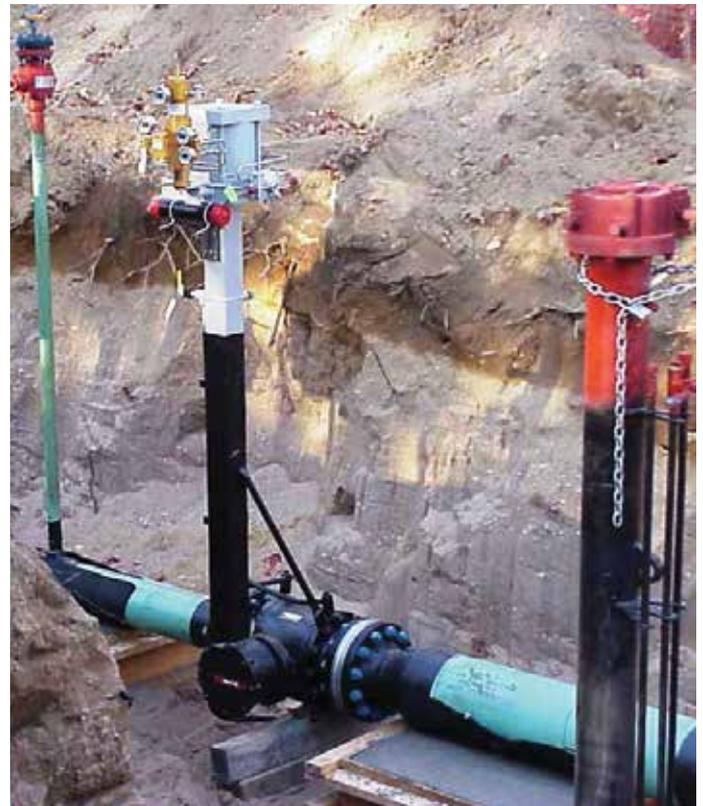
**Figure 2** - Below Ground Ball Valve Regulator combined with Control Valve Silencer.
