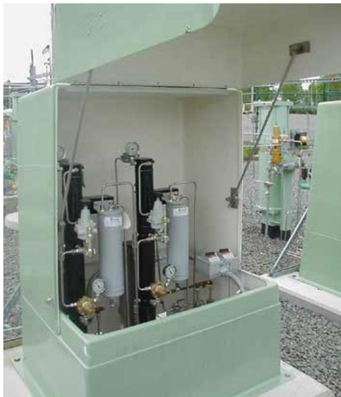
**Figure 4 -** Below Ground Regulator with Fiberglass Cabinet.
