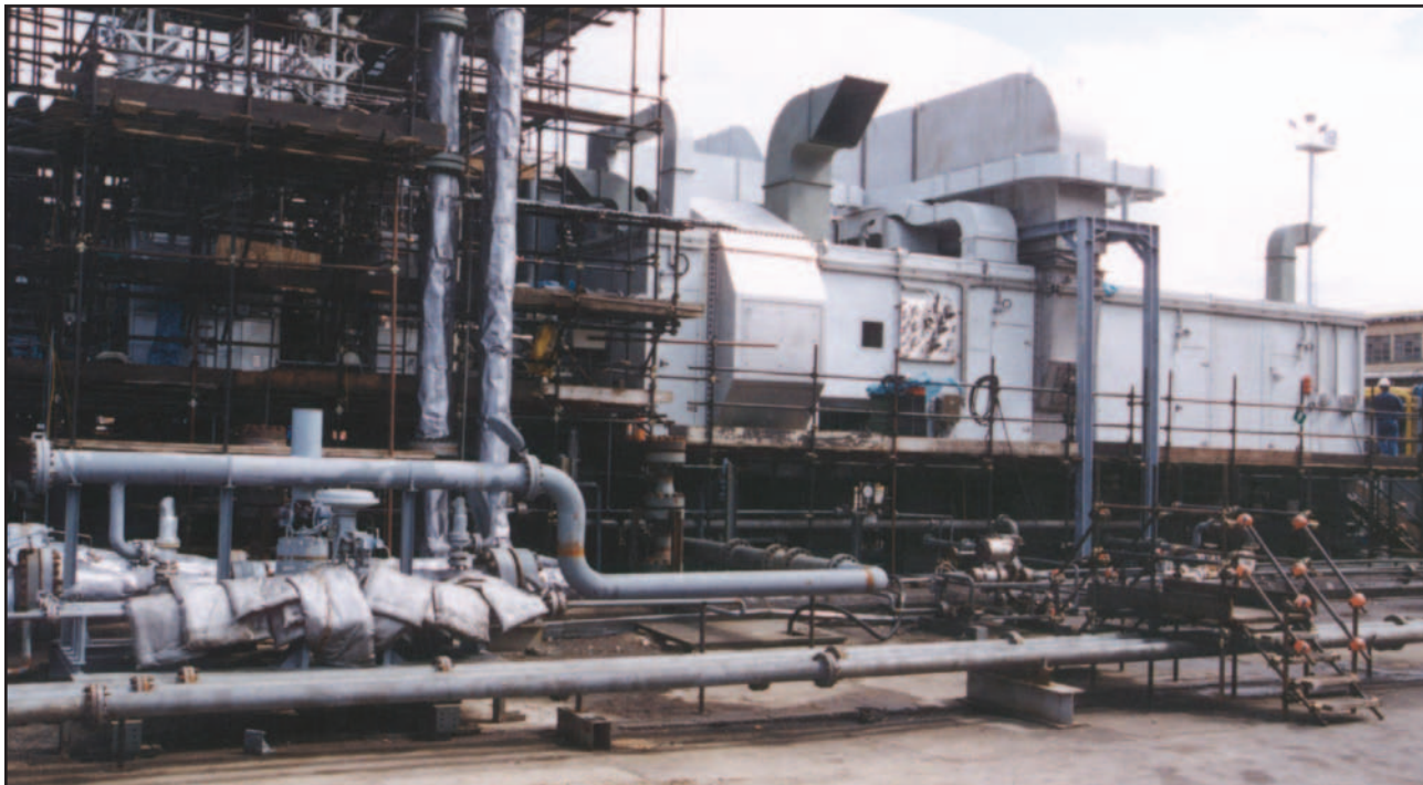
■ One of the Karachaganack sour gas compressor trains during full load test at the Nuovo Pignone Florence shop in 2001. These compressors, similar to the Kashagan ones, have been in service since 2003, with exceptionally high availability and reliability factors.
